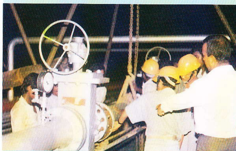
Tie-in work with North-South pipeline at Kailashtilla
