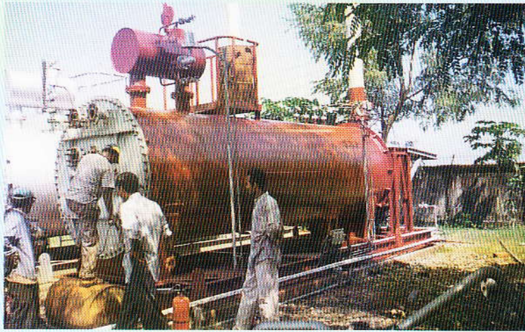
Overhauling works of the Heat Exchanger of 90 MW Power Station at Fenchugonj
